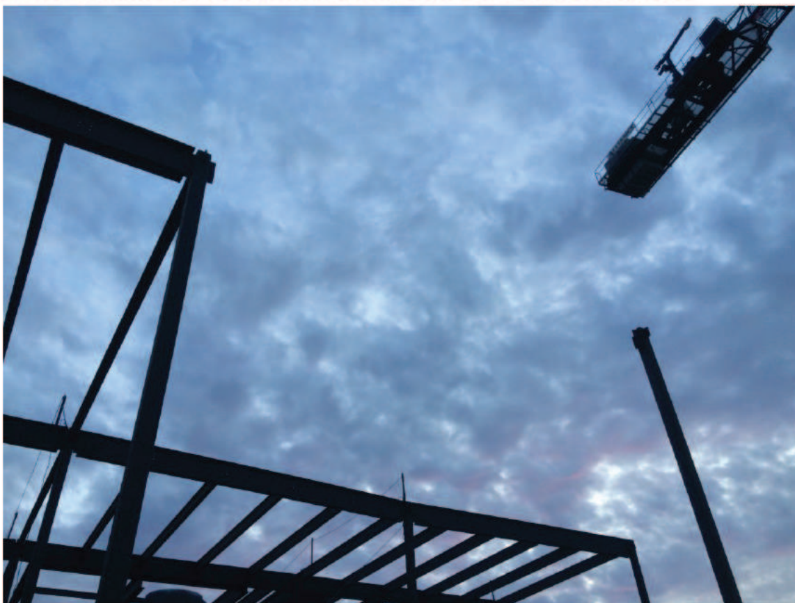
Photo 1: Charpente métallique (source: CNESST)
